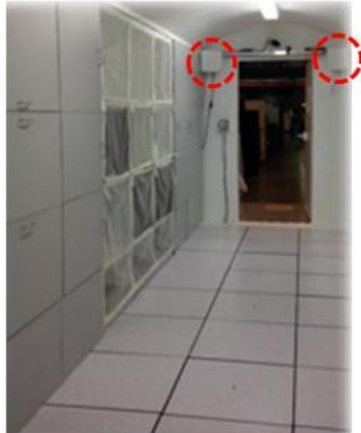
**Figure 6. Red circles mark antennas for the sparse area reader.**
